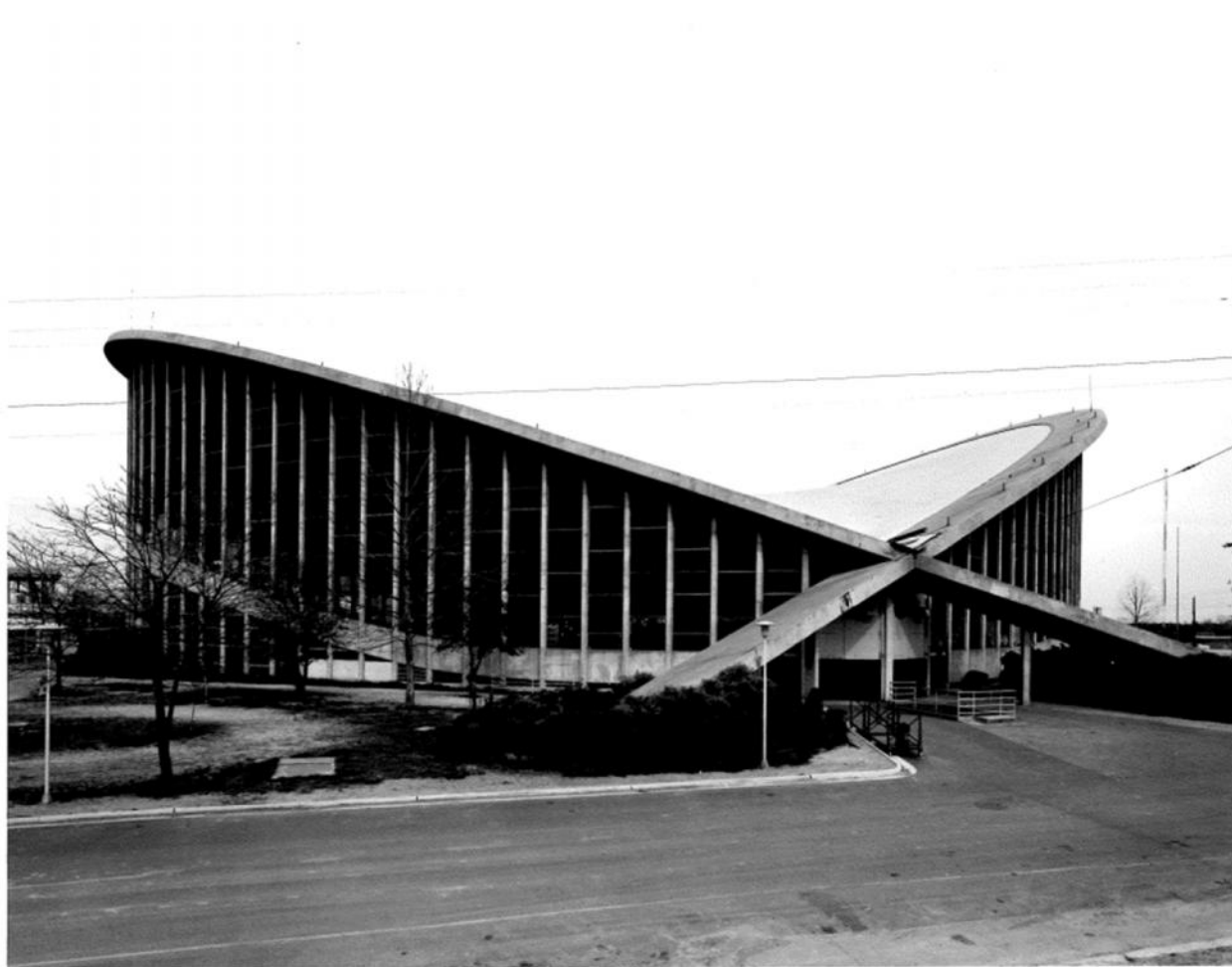
Dorton Arena, 1953. Listed 1972. Photo NC HPO
